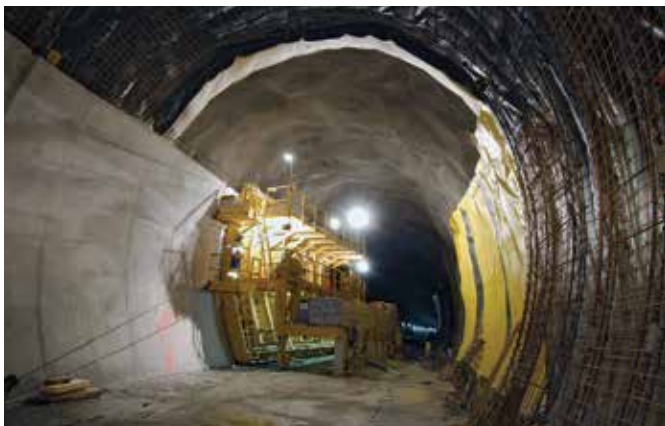
Concrete forms were used for the tunnel's sidewalls, while the roof was sprayed with shotcrete.
