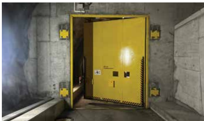
The airlock door swings open after pressurization equalizes, allowing a vehicle to continue down the access road into the tunnel at Mitholz. This would be the route for rescue buses in an emergency.
