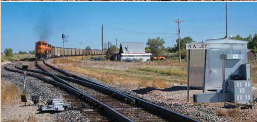
N.A. Junction, east of Pueblo, is the Colorado Pacific's connection with BNSF Railway and the Union Pacific. The connection, previously cut when the line was cast off (top), was reconstructed (bottom) by 2021. The project added 2,700- and 7,600-foot long sidings, enabling the exchange of 110-car unit trains. Three photos, J. L. Gattis
