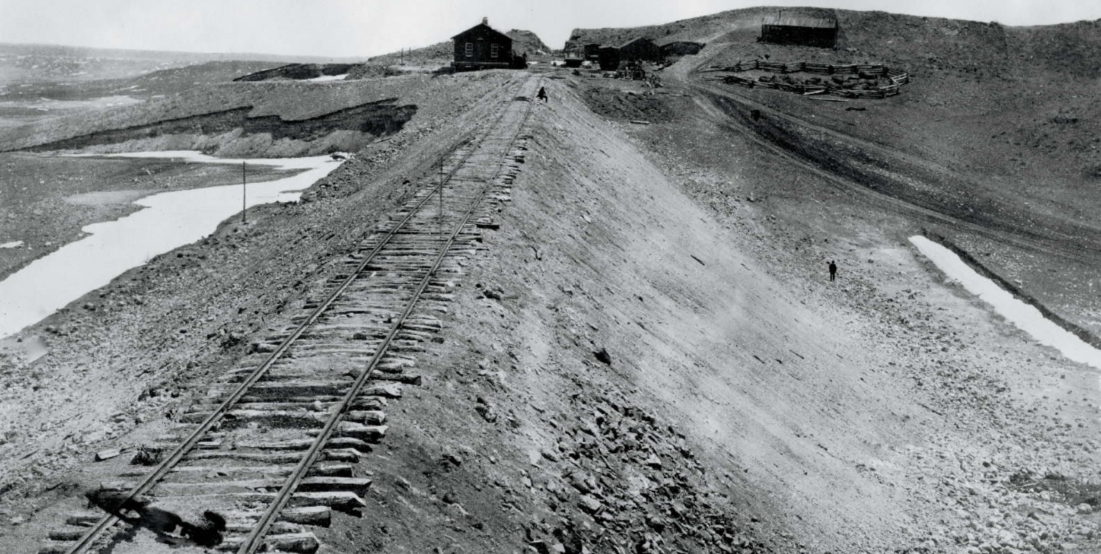
Roadbed and track construction on the original Union Pacific main line was fast and rudimentary. This scene in Wyoming shows the cut-and-fill work, as well as the lack of ballast and the rough-hewn ties that marked the initial effort at building a transcontinental railroad. A.J. Russell
