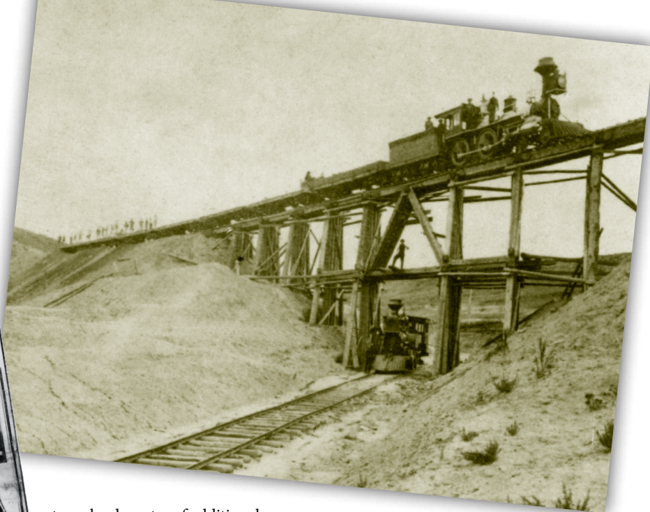
UP crews built a switchback to reach a tunnel during the construction. The work was amazing in many ways. UP
