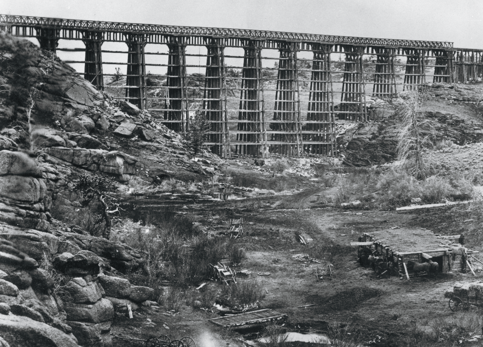
Dale Creek trestle, measuring 650 feet long and 126 feet high, was built during winter 1867-68 using timbers from Chicago. Union Pacific
