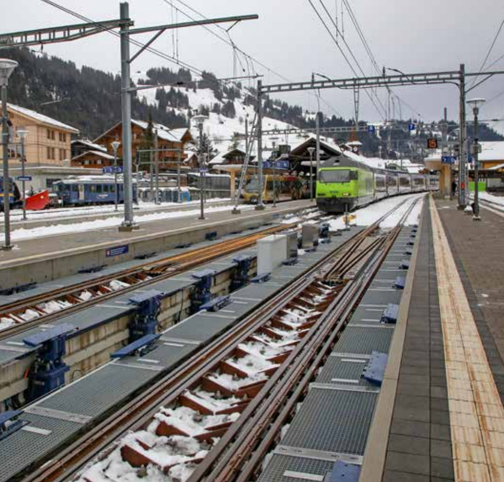
The GoldenPass Express runs through this section of track in Zweisimmen for its wheelsets to make the transition between standard and meter gauge. Keith Fender
