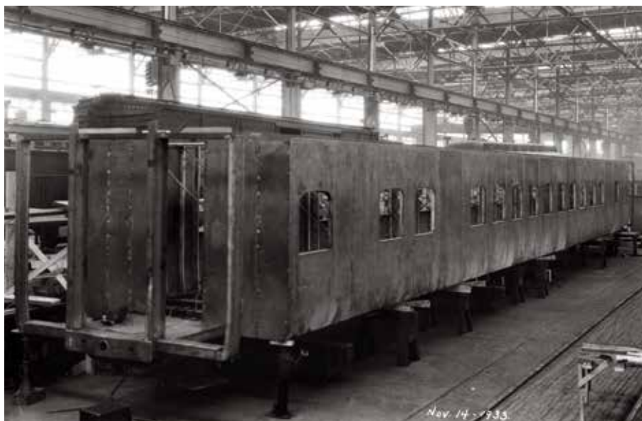
Coach 4400 is under construction at Milwaukee Shops in 1933. This was the prototype for forthcoming lightweight, streamlined passenger cars. Milwaukee Road Historical Association collection
