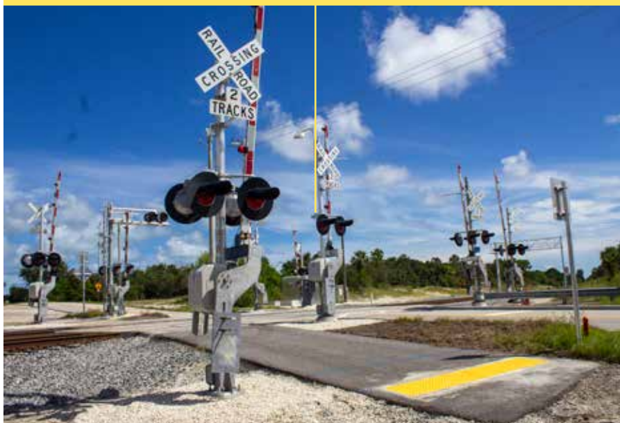
Nine highway warning devices were installed at the rural Walton Road crossing north of Stuart, Fla. The forest of signals includes quad gates for vehicles, pedestrian gates, and radar detection devices.
