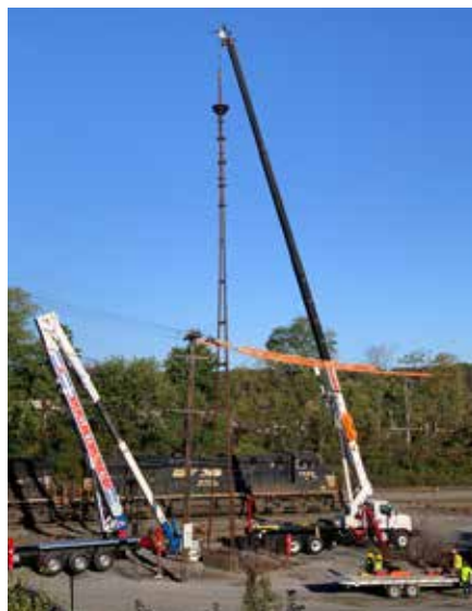
To remove the light towers, NS retained contractor Chris Dell. Dismantling the structures was complicated by proximity to live tracks, overhead power lines, and access within the Altoona, Pa., yard. L.R. Myers
