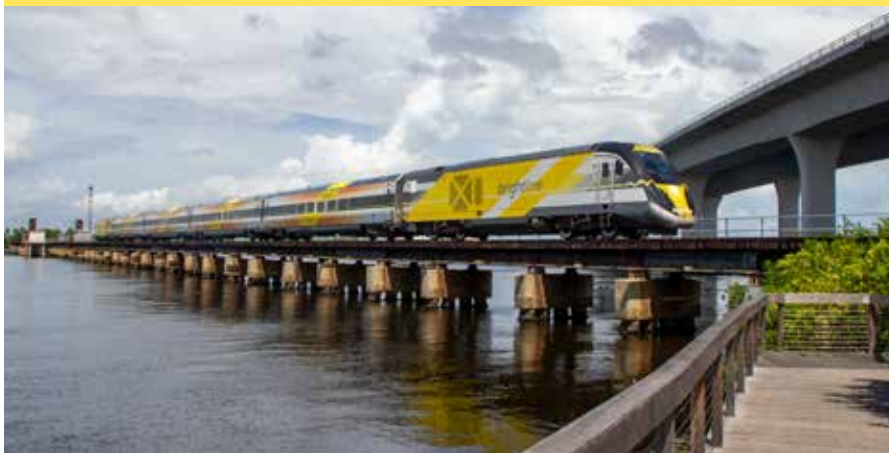
A BrightOrange trainset heads south across the St. Lucie River drawbridge in Stuart, Fla., on Sept. 25, 2023. The single-track bridge is an operating bottleneck that is likely to remain a challenge until a new double-track bridge can be built.
