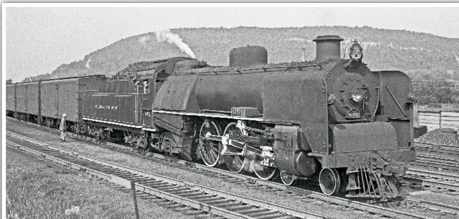
P-1 class Pacific No. 651 handles a passenger train at Whitehall, N.Y., on Aug. 29, 1951. These locomotives were perhaps the most ungainly on the D&H with their smoke deflectors, wide firebox, and long, eight-wheel tender. David T. Mainey, Center for Railroad Photography & Art collection
