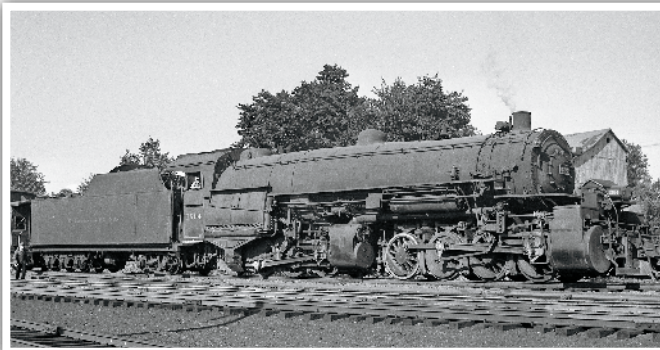
H class No. 0-8-8-0 1604 works in pusher service at Ararat, Pa., on July 14, 1951. D&H President Leonor F. Loree brought the Mallet design with from the B&O. David T. Mainey, Center for Railroad Photography & Art collection
