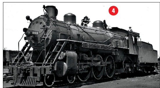
Rock Island 4-6-2 No. 914 was one of 50 class P-33 Pacifics, built by Alco in 1910. Eleven were oil burners, including 914. Robert Graham,
