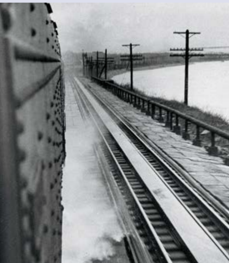
The 6009 takes water on the fly from the track pans at Tivoli, right beside the Hudson River. Experiments with overflow vents and scoop design led NYC to develop equipment that enables water to be taken at up to 80 mph.
