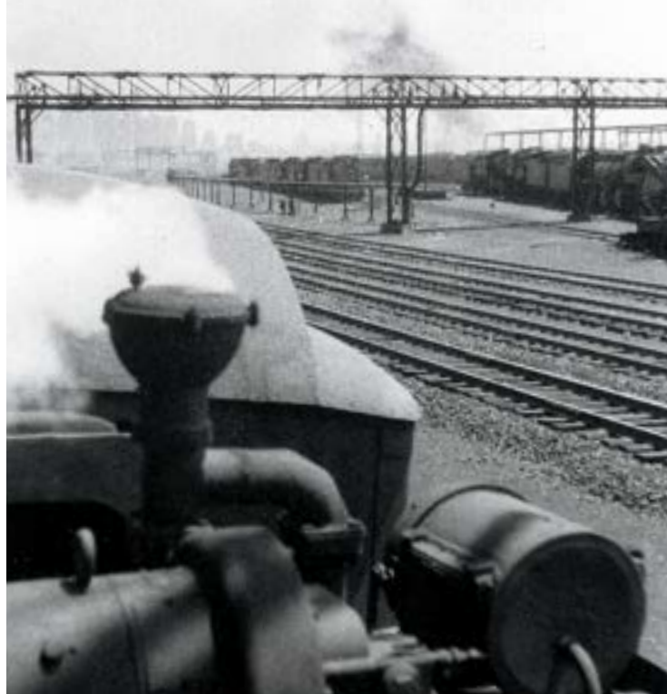
As the train departs Jersey City, a rearward view over the tender headlight and coach-lighting generator shows dead steam engines stored on tracks outside the terminal. Most would never run again.
