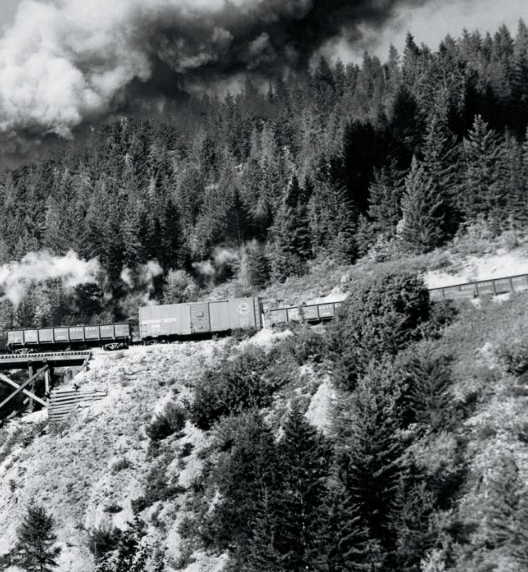
Northern Pacific's branch line from St. Regis, Mont., to Wallace, Idaho, included Lookout Pass, a crossing of the Bitterroot Mountains whose steep grades limited compound 2-8-8-2s to a mere 600 tons. Class Z-3 No. 4020 (Alco, 1920) has just seven cars behind her tank as she fights up the 4 percent climb on the curved trestle just east of Dorsey, Idaho, on September 17, 1953 — not long before diesels arrived. Henry R. Griffiths Jr., Jim Griffiths collection
