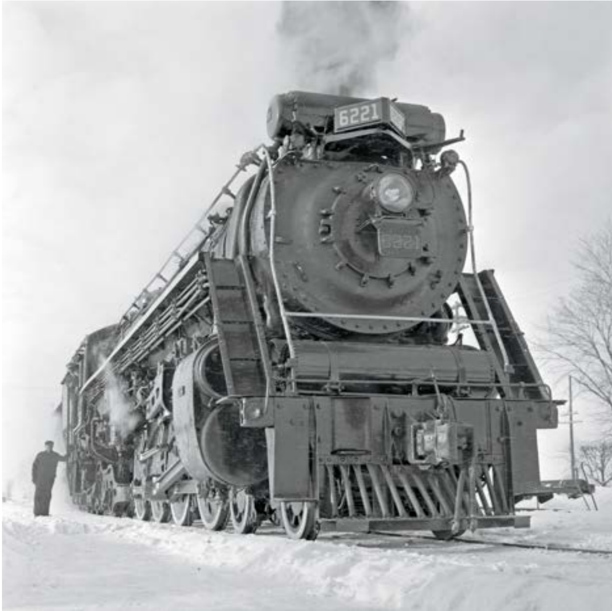
Canadian National 4-8-4 No. 6221 pauses at Sebringville, Ontario, during a test run after being overhauled in the "Big Shop" at nearby Stratford. The date is January 8, 1959, and the Northern type is one of Stratford's last major jobs. As CN's last steam repair facility, Stratford was one of the final pieces of steam's North American empire to crumble. James A. Brown
