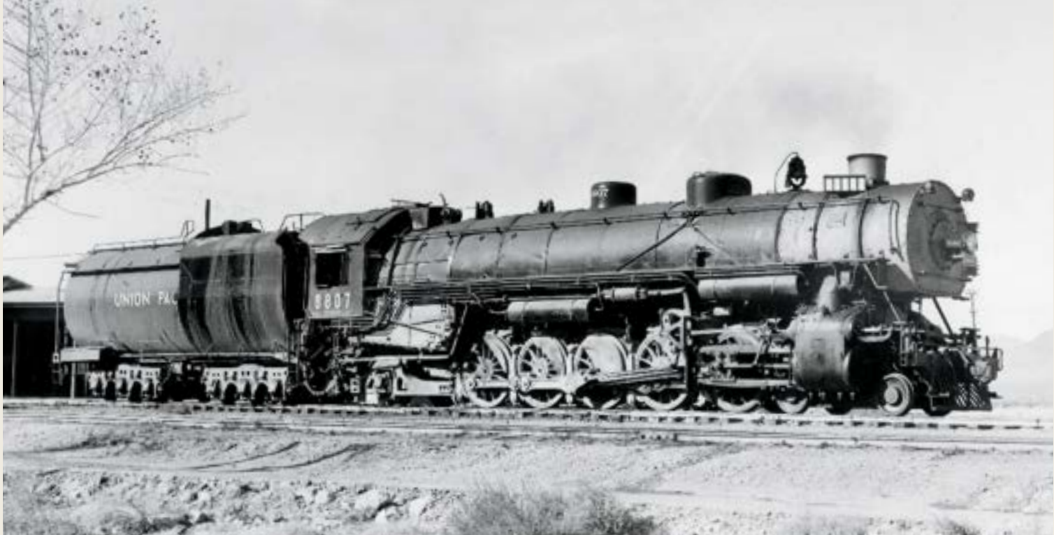
Three-cylinder 4-10-2 No. 8807 shows off its long lines at Yermo in late 1939; Thrall fired sister 8800 west from here in March '41. There were 60 4-10-2s built, all three-cylinder, all during 1925-27; SP and UP had 49 and 10, respectively (all from Alco), and Baldwin built one as a demonstrator, which was never sold.
