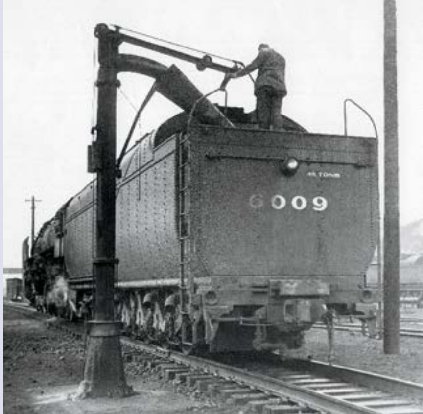
The Niagara's 18,000-gallon centipede tender is topped off with water. Next stop: the coal wharf.
