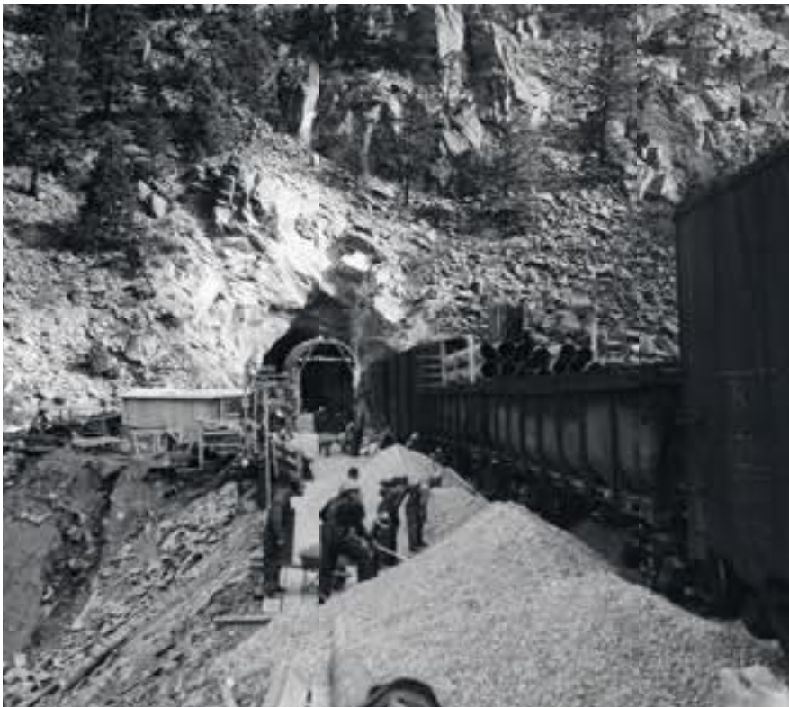
Men are busy shoveling gravel as cars filled with material arrive at Tunnel 10's west portal. Workers from a nearby water tunnel construction project assisted railroad crews.
