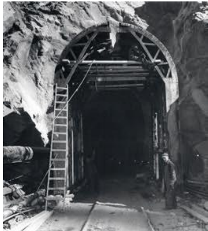
Workers erected a steel arch framework at the western entrance to the fire-damaged 1,570-foot tunnel.
