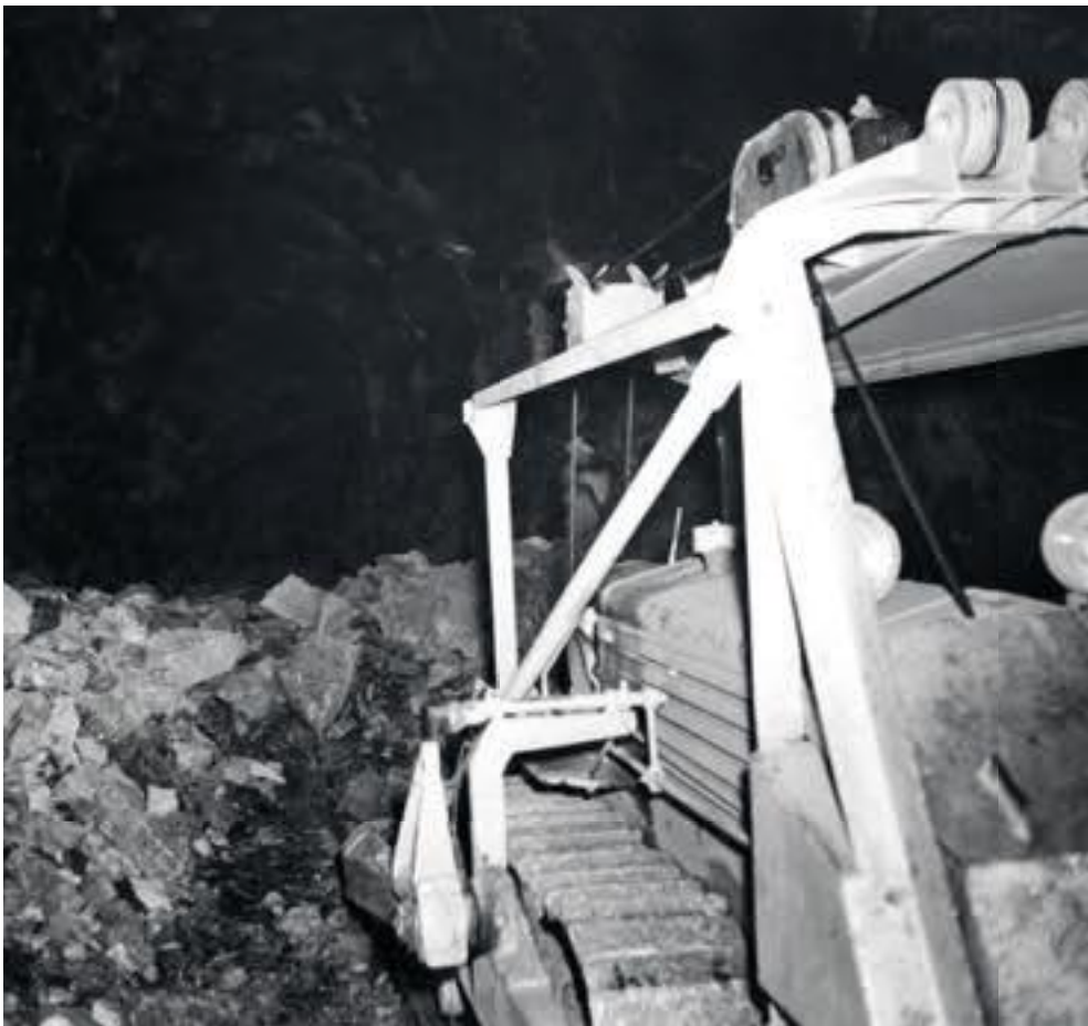
Bulldozers "mucked out" tons of loose rock in the burned portion of the tunnel. Note the rock that was charred by the tremendous heat in the crown of the bore.
