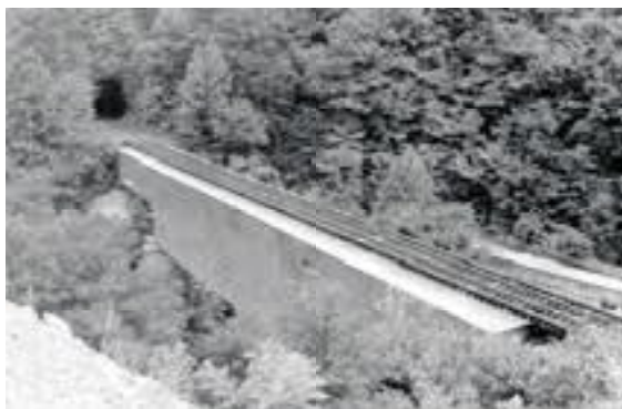
Just west of Hampton, ET&WNC crosses the Doe River on a deck-truss bridge whose structural members are covered, then goes right into one of the line's several tunnels.
