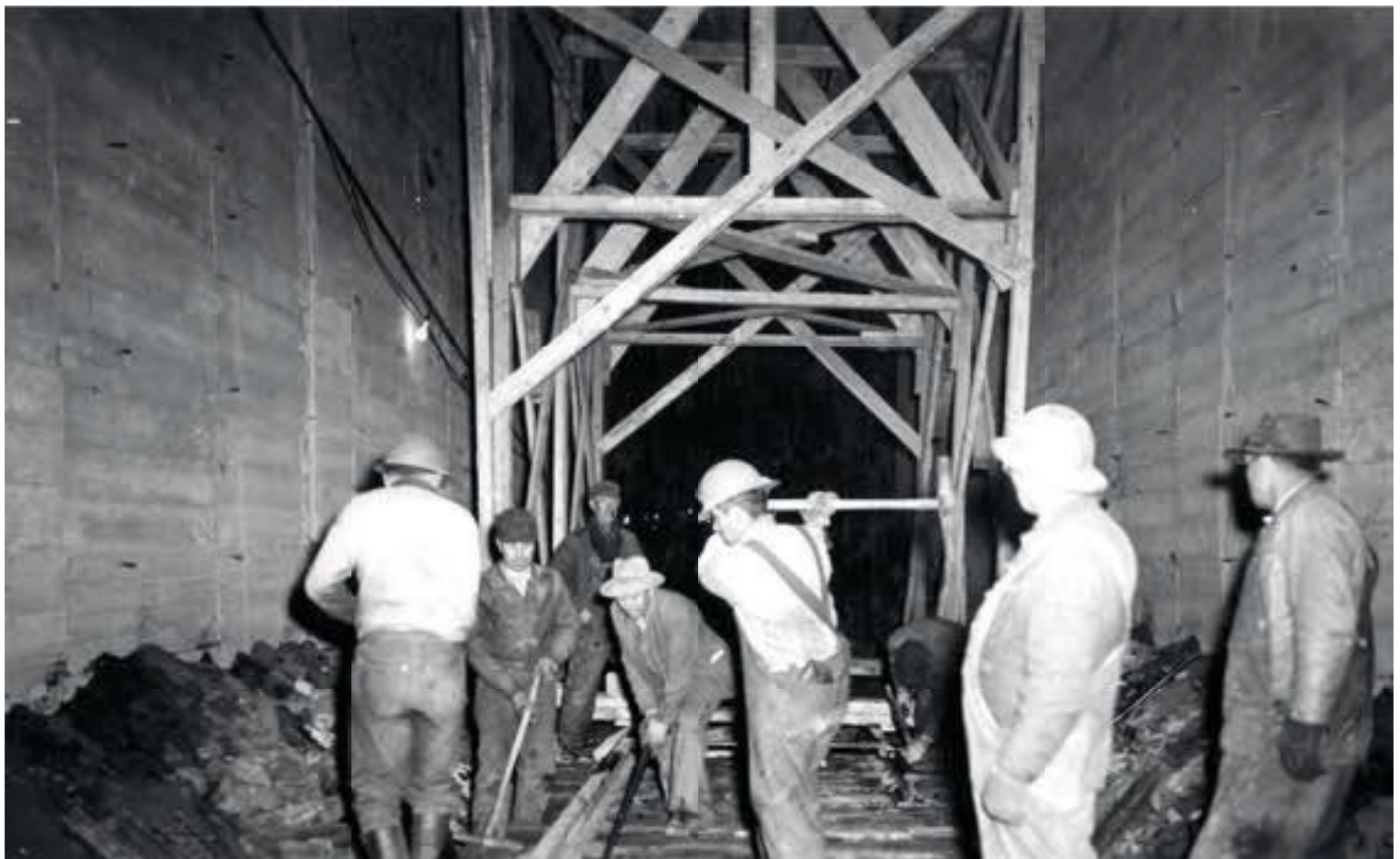
With the concrete lining in place, but some wood framing and rock yet to be removed, track crews spike down new steel inside the tunnel. Thousands of miles from the front lines, these men are doing their part for the war effort.
