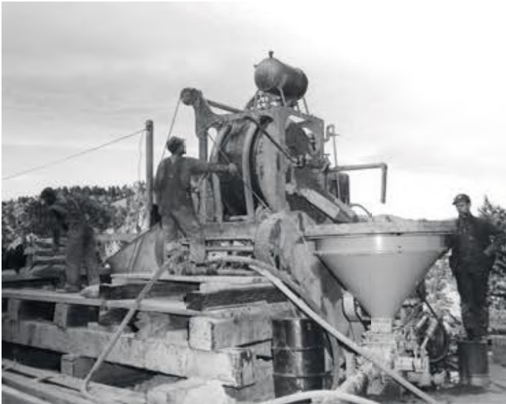
Concrete mixers mounted on improvised platforms (above) provided material for the tunnel's new lining. Portable generators (below) supplied electricity for the mixers and other equipment.
