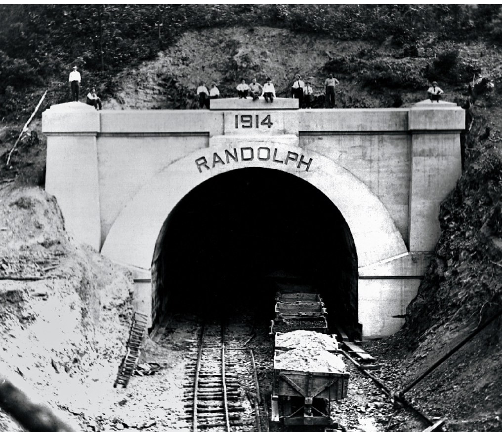
Work on the Magnolia Cutoff began in March 1913, and as the date on the west portal of the nearly completed Randolph Tunnel indicates, progressed rapidly. Tunnels were lined with brick to protect them from damaging steam locomotive exhaust.
