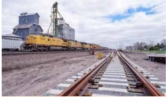
14:58 Just passing by Brady. CB&N-10 passes a prefabricated high-speed turnout at Brady, Neb., 261 miles west of Council Bluffs, Iowa. Scott A. Hartley
