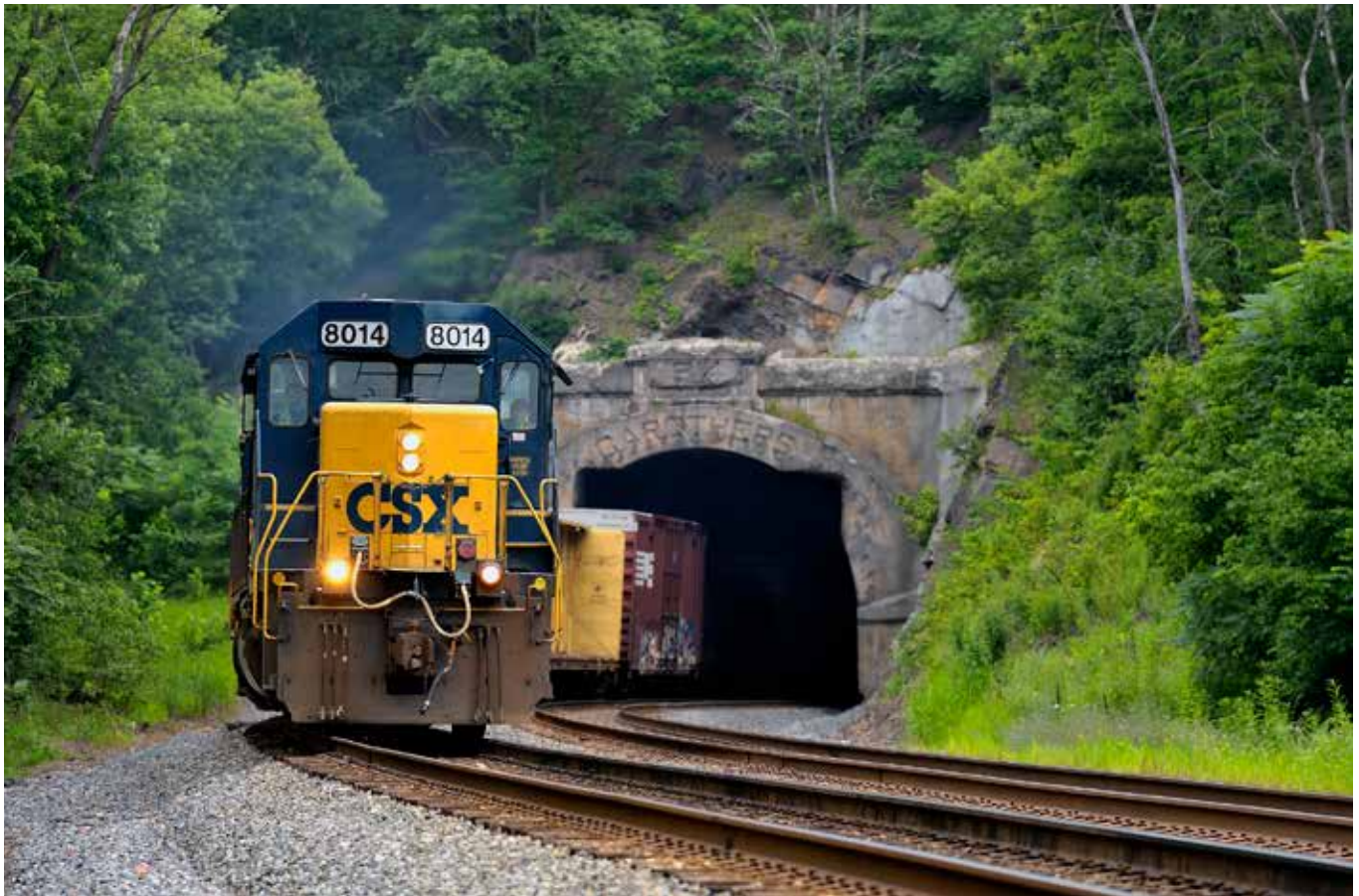
The 993-foot Carothers Tunnel, near the town of Paw Paw, W.Va., is the westernmost of the four bores required for the cutoff. This tunnel needed some 8,000 cubic yards of concrete lining. The notches have created clearance for double-stack traffic.
