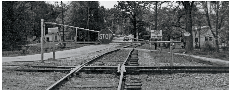
A pipe gate with a stop sign attached protects a crossing between the Ashley, Drew & Northern and Missouri Pacific in Monticello, Ark. Trains on the AD&N had to stop, check for oncoming MP trains, and open the gate before crossing the diamond. Terry
