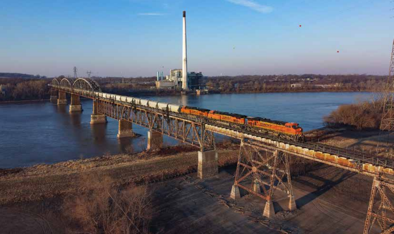
The last great barrier to complete double-tracking of BNSF's Chicago-Los Angeles route is this bridge over the Missouri River at Sibley, Mo., shown in 2012. Construction of a second bridge has begun. Zach Pumphery
