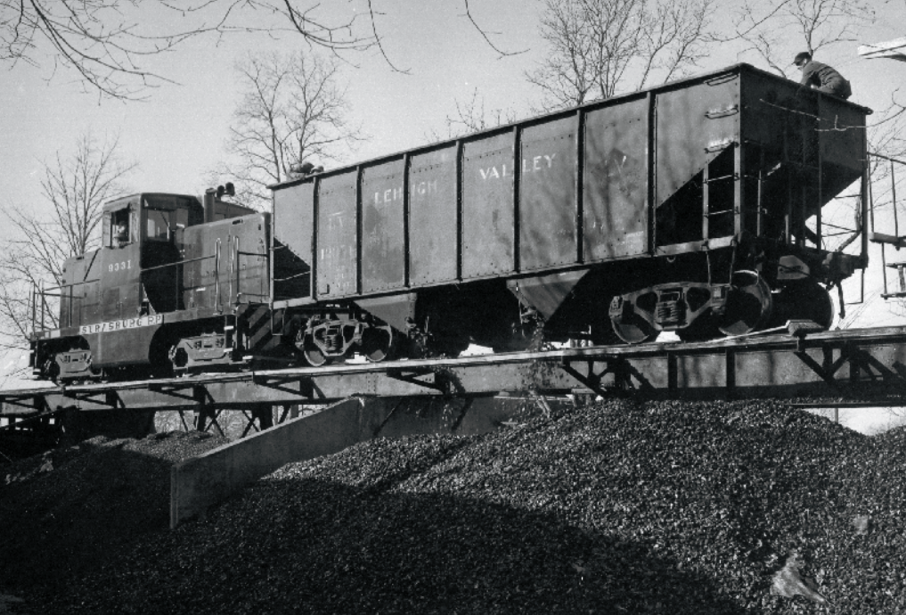
In 1961, leased Pennsylvania Railroad GE 44-ton switcher No. 9331 spots a coal load on the Graybill trestle in Strasburg, Pa. The trestle is now dismantled. The Strasburg Rail Road later bought the unit and relettered it to No. 33. Kurt Bell collection
