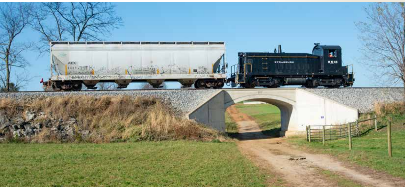
Line improvements were made to handle contemporary freight cars including the 2011 construction of a concrete bridge over the Pumpkinville Turnpike, which is really just a dirt farm path. The design and styling of the new bridge was inspired by a Lackawanna Railroad design.
