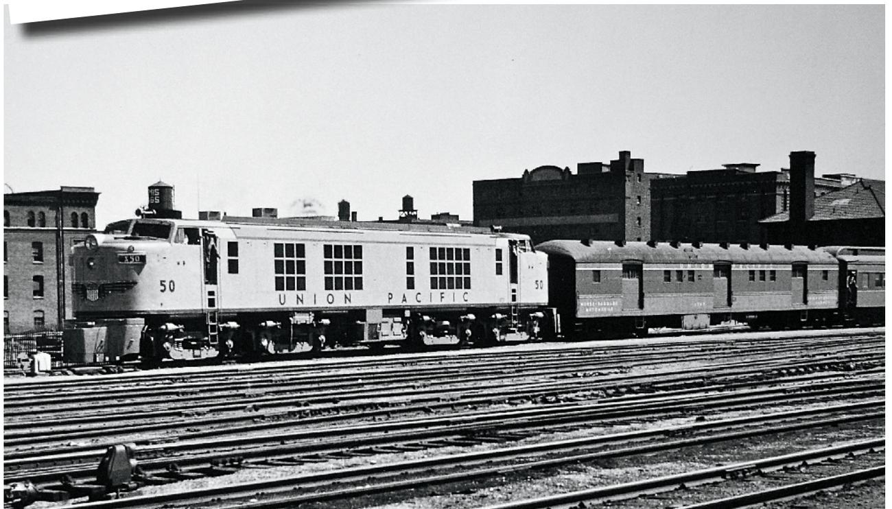
After milling around machine for about an hour, a trainload of dignitaries boarded a westbound extra behind the Union Pacific's new gas turbine electric No. 50. This was an oddball sighting, compared with the myriad of steam and E7 diesels.
