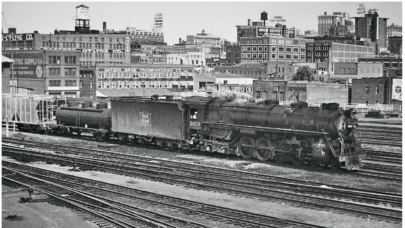
Eastbound Rock Island 4-8-4 No. 5059 moves through the maze of trackage west of the Omaha station with a freight train. The 4-8-4-type was the largest steam locomotive on the Rock's roster, classed R-67B and carrying Nos. 5000-5064 and 5100-5119.
