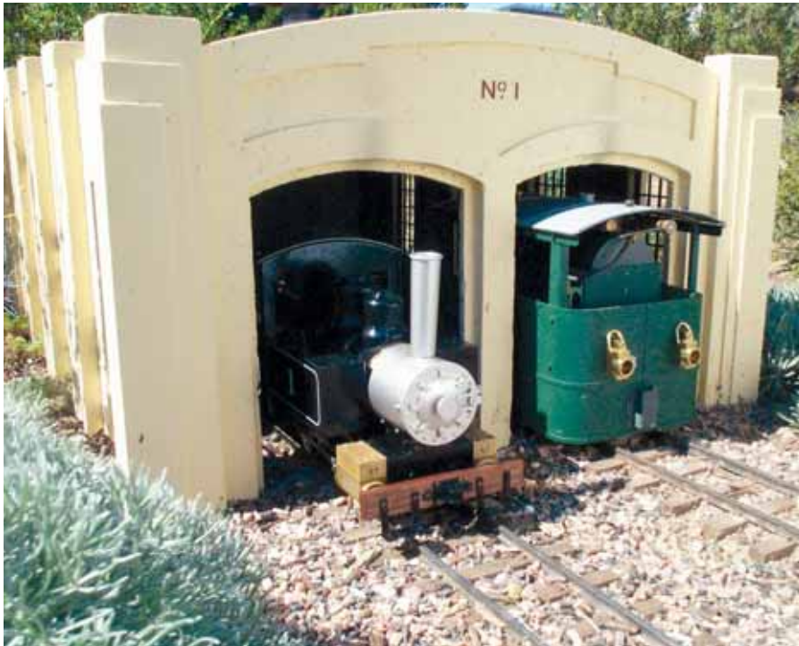
Nothing beats concrete for strength and durability when it comes to buildings. This is a versatile medium that can be used as easily for bridge piers as for engine houses, like this one on Marc and Barb Horovitz's Ogden Botanical Railway.
